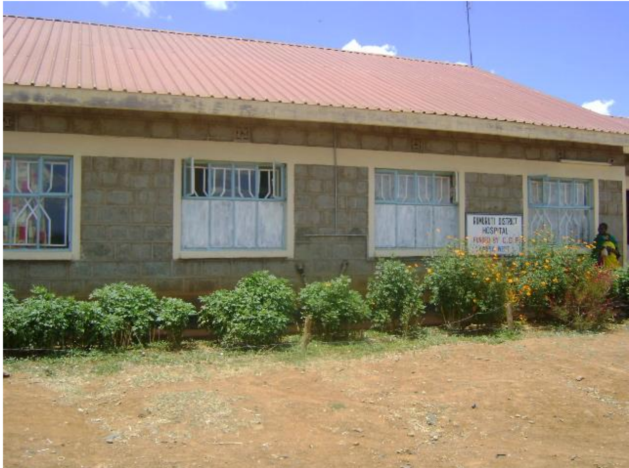
Rumuruti District Hospital
